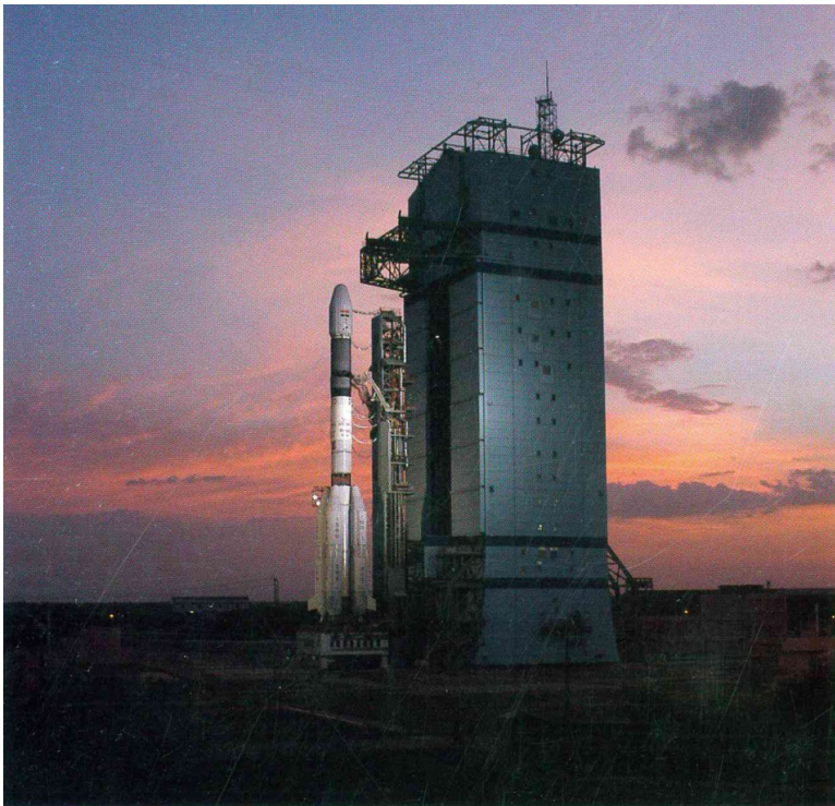
16. A stunning view of the GSLV on the pad, as the sun paints the sky red!
